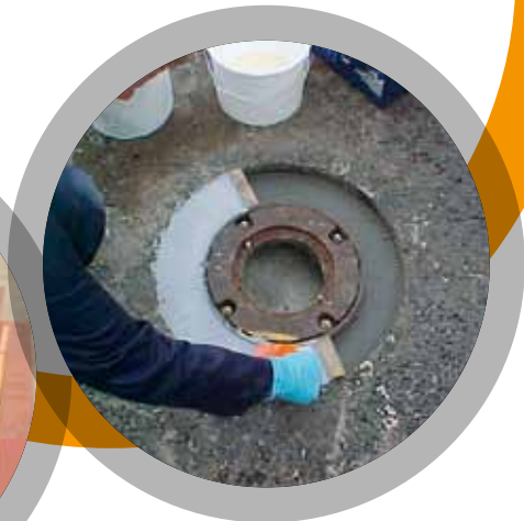
Grouting Runway Lights
